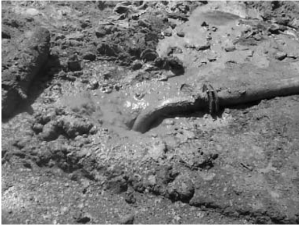
Fig. 2. Grouting works on the DP motorway construction site (photo: R. Jendruś).
