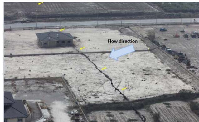
Figure 4. Aerial view of the northern section of the crack (courtesy of Puerto Lumbreras City Council). The yellow arrows indicate the location of the earth fissure (modified from Mulas, 2013).
